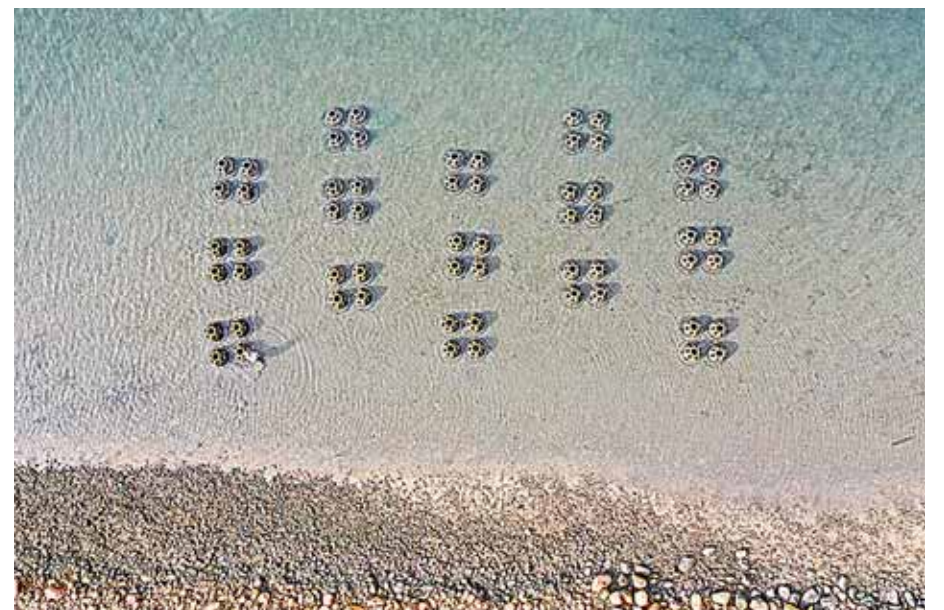
Reef balls, made from a mixture of cement, sand and crushed oyster shells, form the South Bay Native Oyster Living Shoreline Project, are seen near the Chula Vista Wildlife Refuge in Chula Vista, California. —AFP photos
