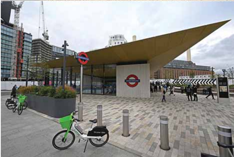
This combination of pictures shows (top) Battersea Power Station underground station under construction near to Battersea Power Station in south London and (down) Battersea Power Station underground station near to Battersea Power Station in south London on October 14, 2022. — AFP photos
