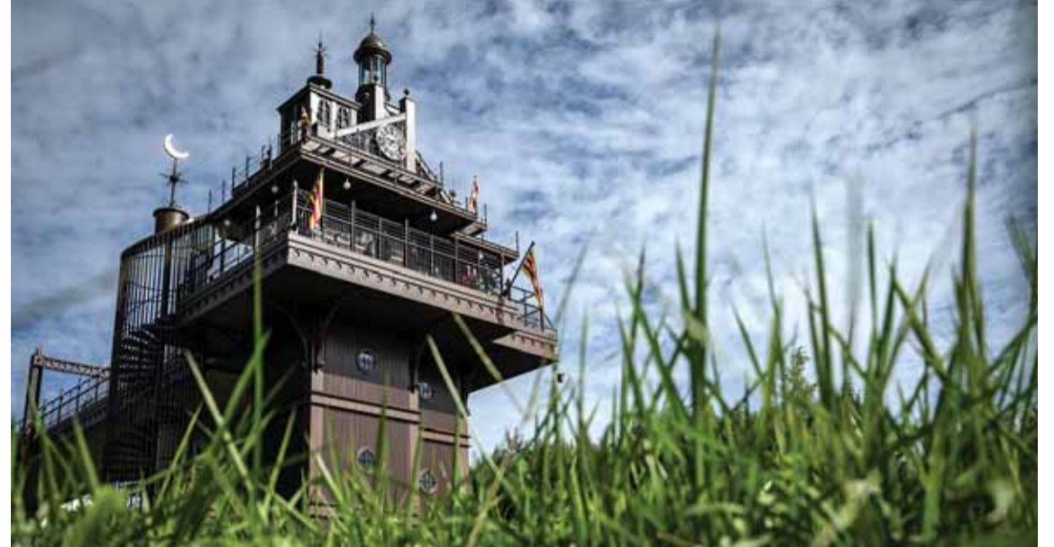
An elevator tower is seen during a media tour of the new Ghibli Park.
