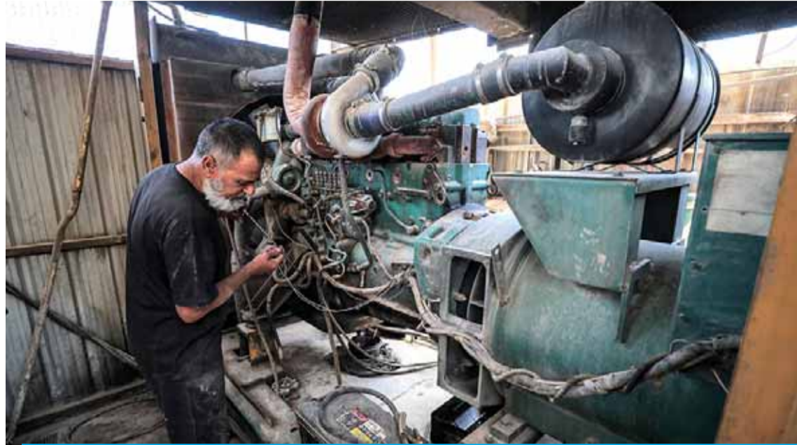
SADR CITY, Iraq: A technician checks the oil on the dipstick of one of the fuel-based electricity generators in the eastern Sadr City suburb of Iraq's capital Baghdad. — AFP
