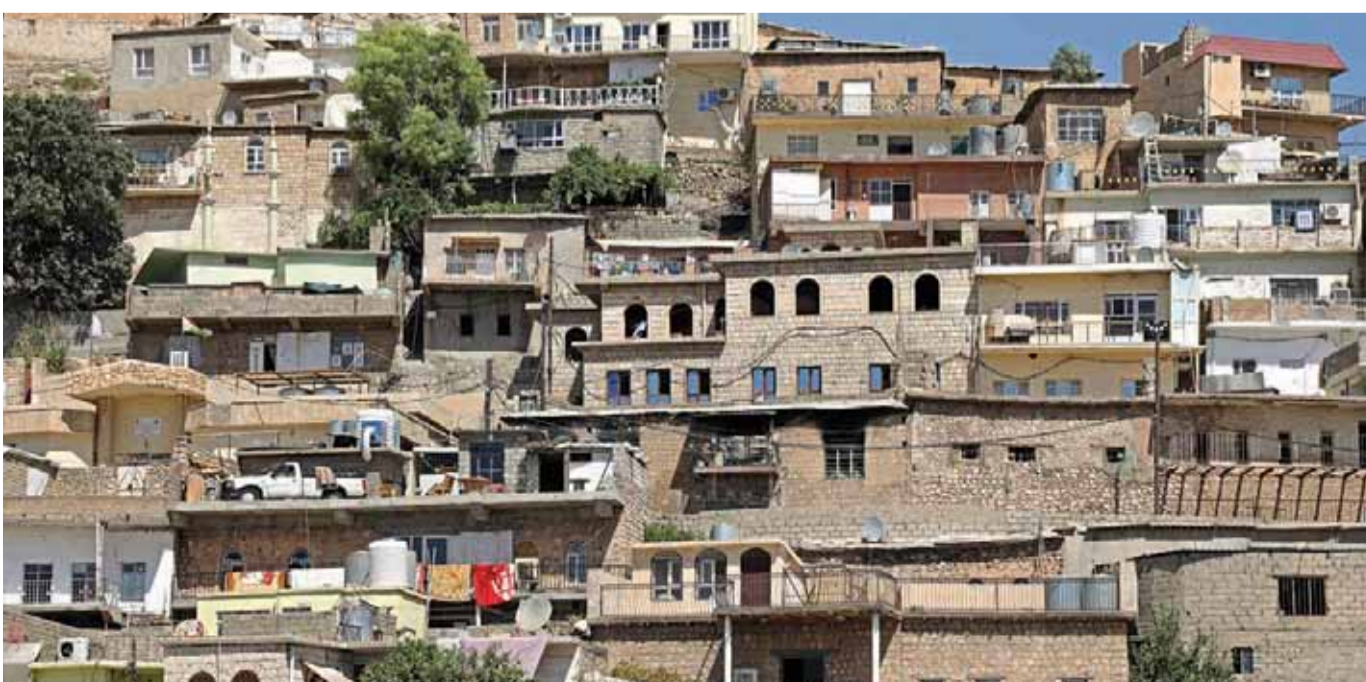
A partial view shows houses in the Kurdish town of Akre, 500 kilometers north of Iraq's capital Baghdad. Concrete houses are nearly everywhere in Iraq, but the northern city of Akre likes to do things differently, opting for stone instead, reaping benefits in the fight against climate change. — AFP photos
