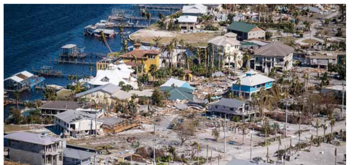
FORT MYERS BEACH, United States: An aerial picture taken on September 30, 2022 shows destroyed houses in the aftermath of Hurricane Ian in Fort Myers Beach, Florida. —AFP
