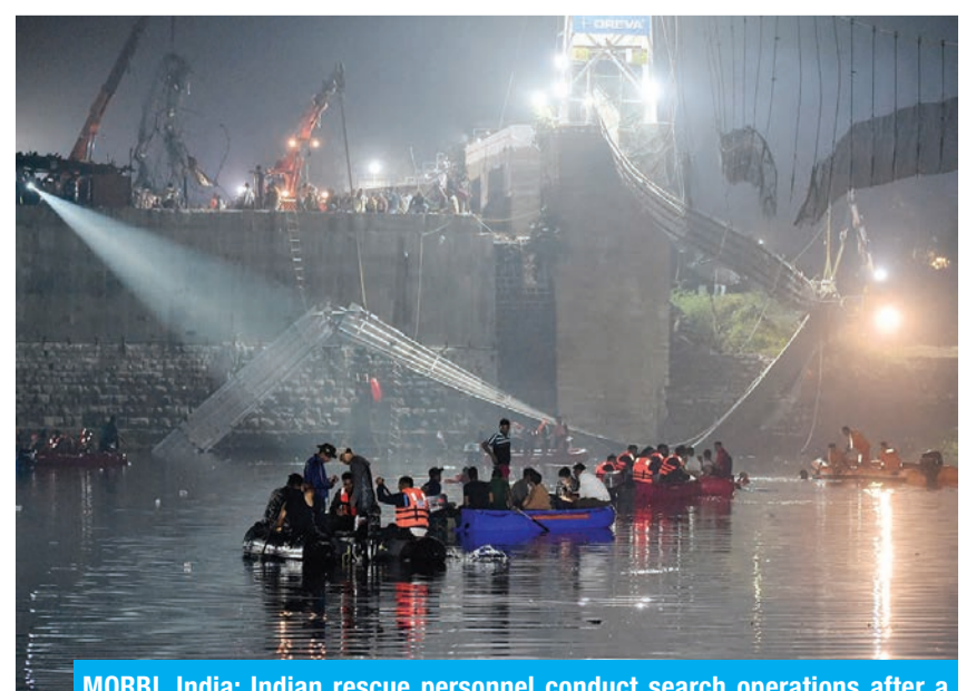
MORBI, India: Indian rescue personnel conduct search operations after a bridge across the river Machchhu collapsed on Oct 31, 2022. — AFP
