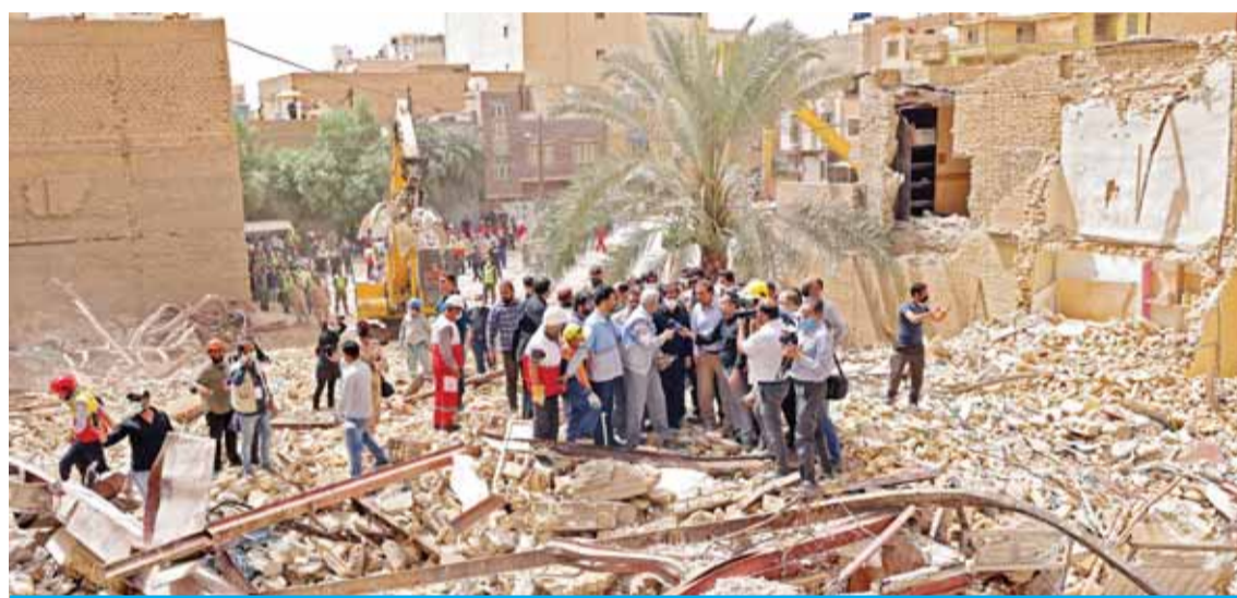
ABADAN, Iran: Handout picture shows Iranian vice president Mohammad Mokhber (C) visiting the site where a ten-storey building collapsed in the southwestern city of Abadan on May 27, 2022. —AFP
