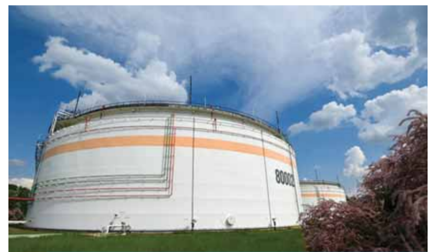
A fuel tank at the Duna (Danube) Refinery of Hungarian MOL Company near the town of Szazhalombatta, about 30km south of Budapest. The Duna refinery continues to receive Russian crude through the Druzhba pipeline. —AFP
