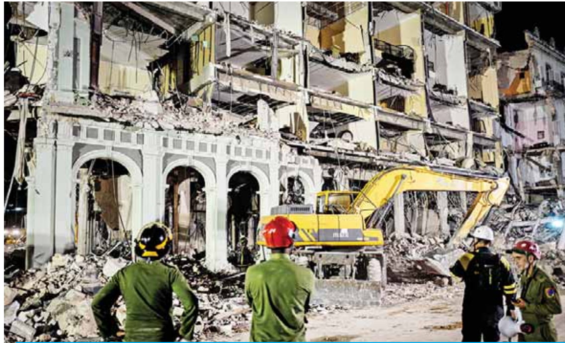
HAVANA: Firefighters and rescue workers remove debris from the ruins of the Saratoga Hotel, in Havana. The death toll from a powerful explosion at a five-star hotel in central Havana climbed to 25 with more than 50 people injured after a suspected gas leak, according to official tallies. — AFP
