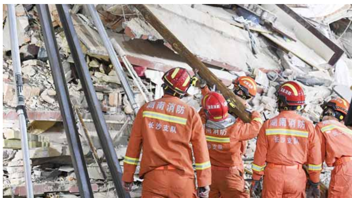
CHANGSHA, China: Photo shows rescuers searching for survivors at a collapsed six-storey building in Changsha, central China's Hunan province. Dozens of people were trapped under a building which collapsed in central China, officials said. —AFP
