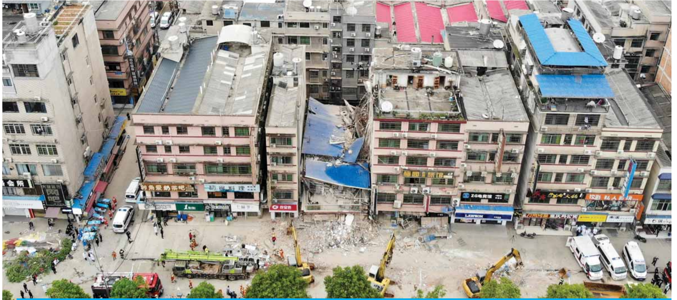
CHANGSHA: This aerial photograph taken on April 29, 2022 shows rescuers working after a six-storey building collapsed in Changsha, in China's central Hunan province. —AFP
