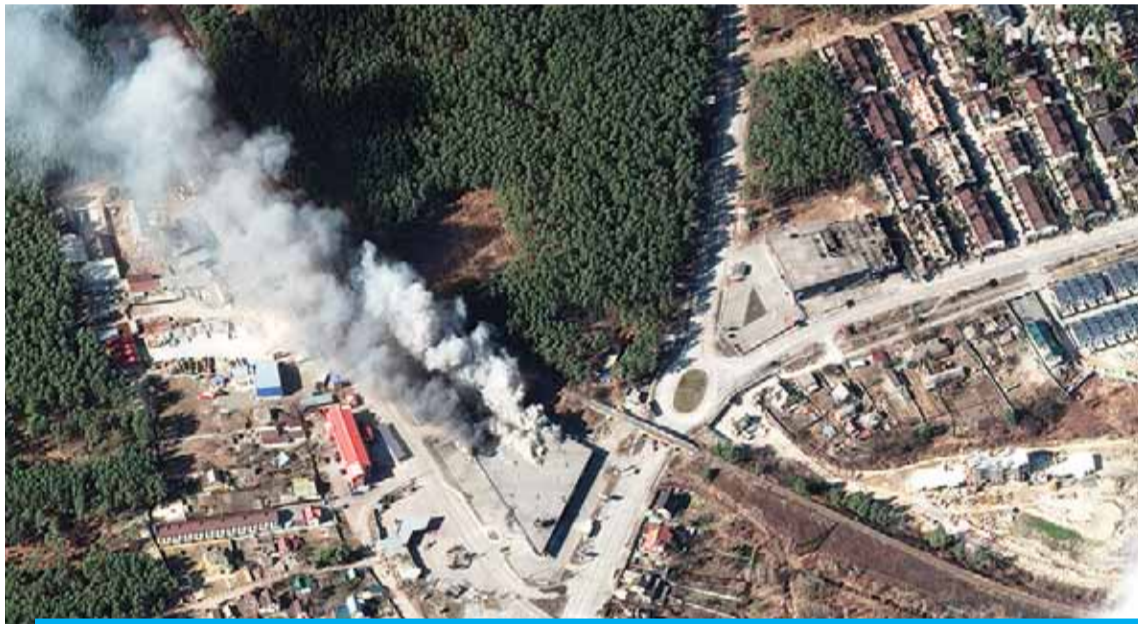
HOSTOMEL, Ukraine: This handout picture released Friday by Maxar satellite image shows a burning city market grocery store and damaged residential buildings, in Hostomel northwest of Kyiv. — AFP
