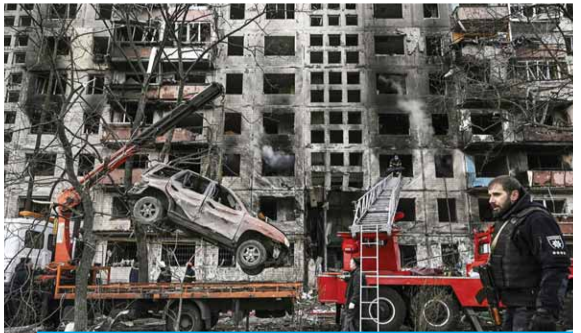
KYIV: A crane removes a wrecked car from in front of a destroyed apartment building after it was shelled in the northwestern Obolon district of the Ukrainian capital yesterday. — AFP
