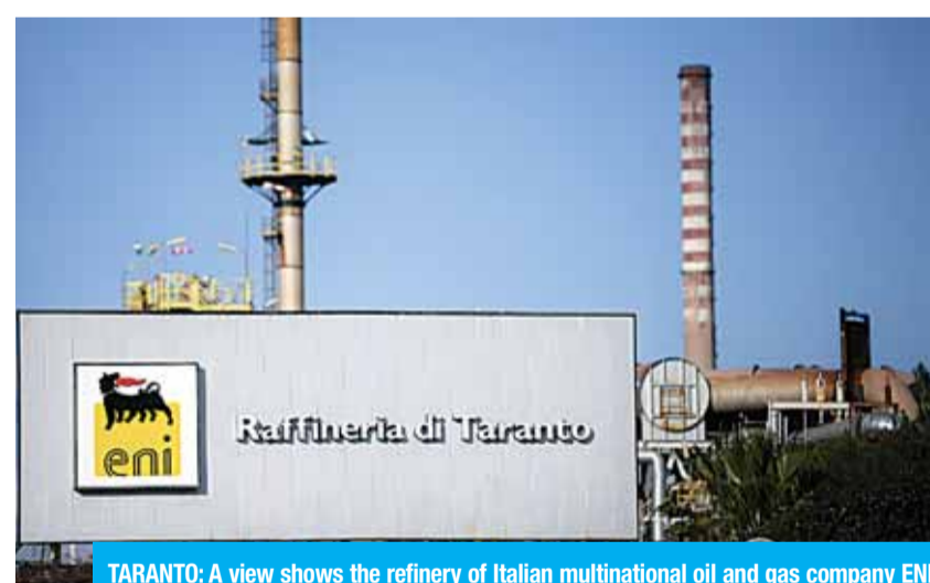
TARANTO: A view shows the refinery of Italian multinational oil and gas company ENI on March 9, 2022 in Taranto, southern Italy. —AFP
