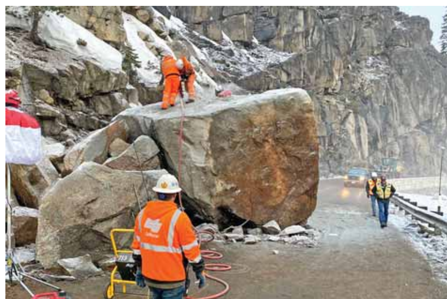
In this handout image courtesy, a big boulder blocks US route 50 as crews work in the area, at Echo Summit near Lake Tahoe, California. — AFP
