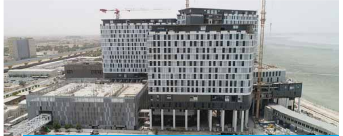
KUWAIT: The New Maternity Hospital Project in Al-Sabah medical zone.
