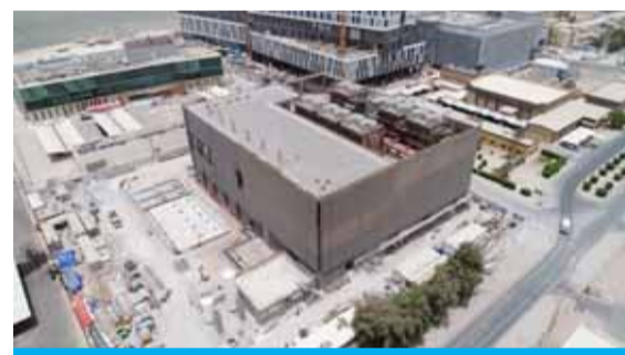
The generator building of the hospital.
