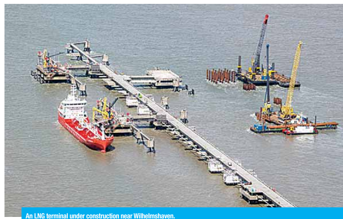
An LNG terminal under construction near Wilhelmshaven.
