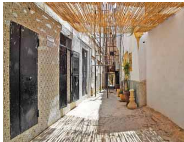
A damaged building in the Casbah of Algiers.—AFP photos
