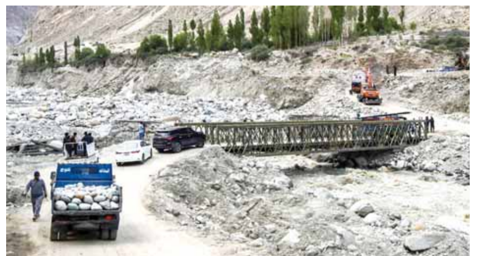
In this picture taken on June 9, 2022, locals and tourists drive through a temporary bridge after the main bridge was swept away by a lake outburst because of a melting glacier, in Hassanabad village of Pakistan's Gilgit-Baltistan region.
