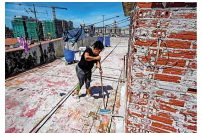
A woman sweeps the floor in a building at risk of collapse in Havana.
