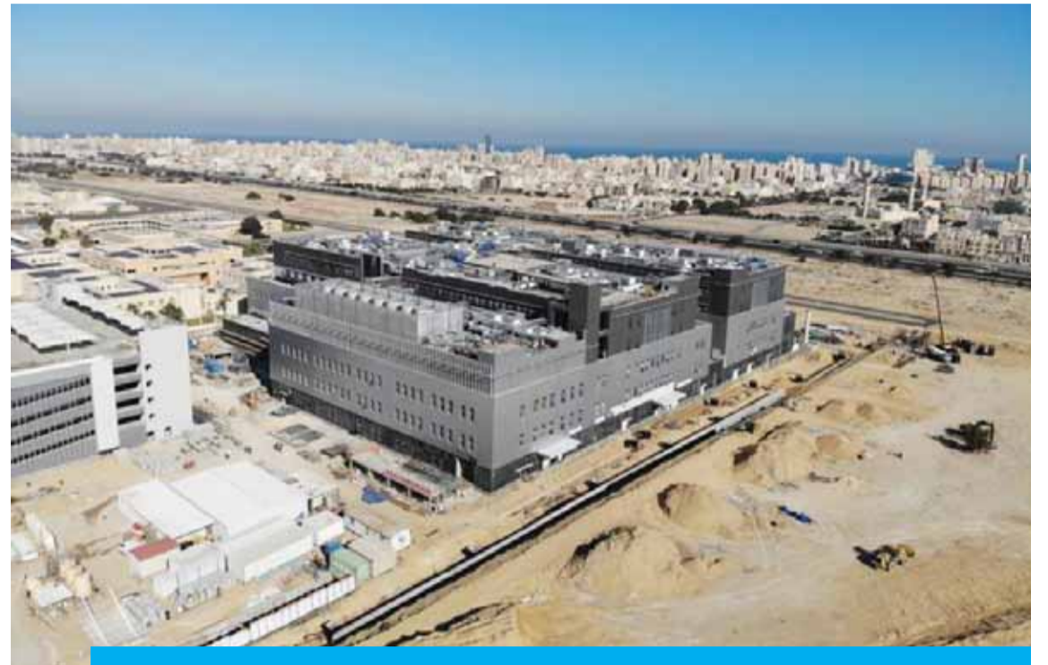
KUWAIT: One of Dhaman's hospitals under construction. —KUNA
