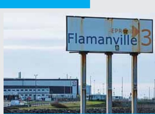
EDF is building its first EPR, a technology that heats highly pressurized water to power a steam turbine, at Flamenville in northwestern France.
