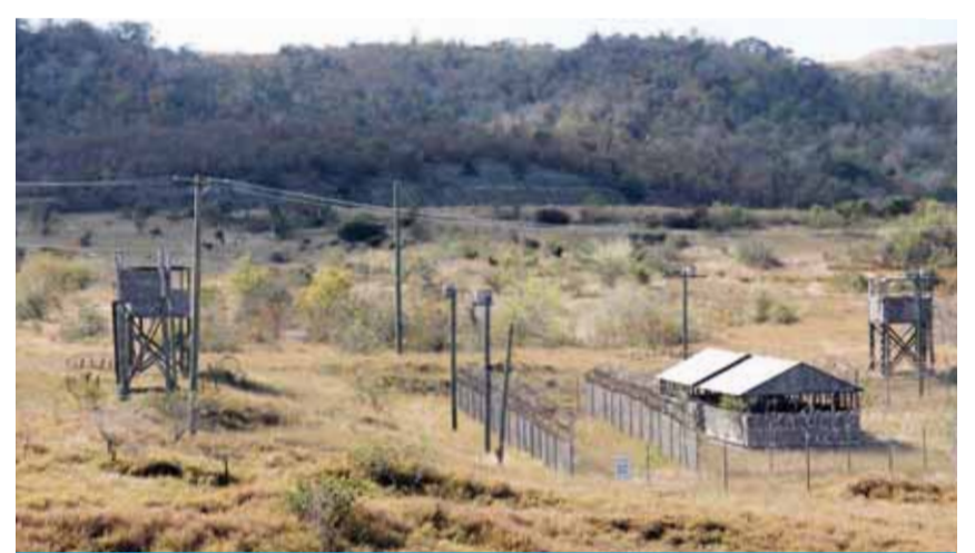
GUANTANAMO BAY NAVAL BASE, Cuba: In this file photo taken on January 27, 2017 the long-abandoned military detention center Camp X-Ray is seen at Guantanamo Bay. —AFP
