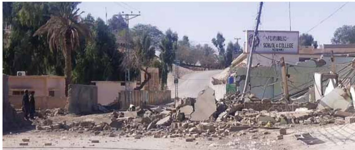
NUSHKI, Pakistan: Security personnel (L) stand beside a destroyed security post following overnight attacks by militants on security camps in Naushki district of Balochistan province yesterday. — AFP
