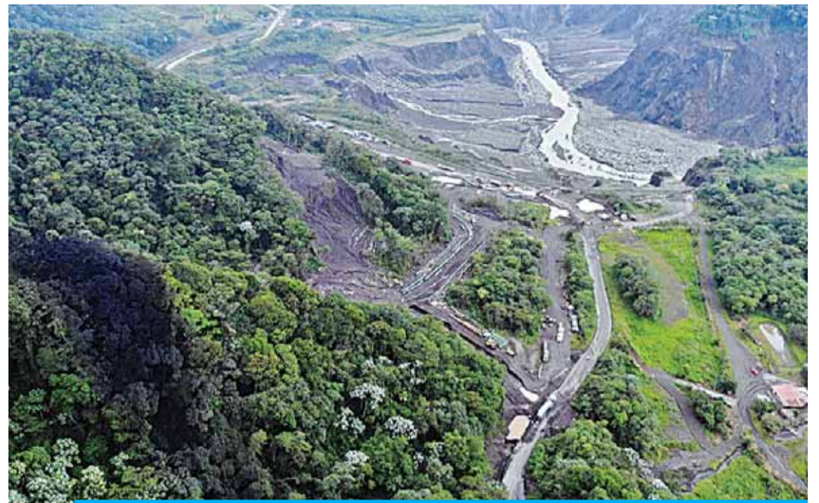
PIEDRA FINA, Ecuador: Aerial view of a sinkhole and the oil spill in Piedra Fina, Amazonian province of Napo, Ecuador on January 31, 2022.
