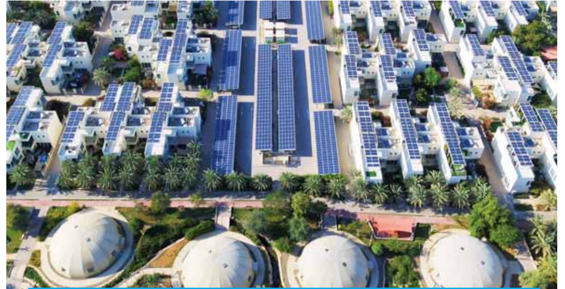
The solar panels are seen on top of the houses.
