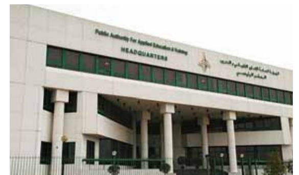
The Public Authority for Applied Education and Training (PAAET) Headquarters.
