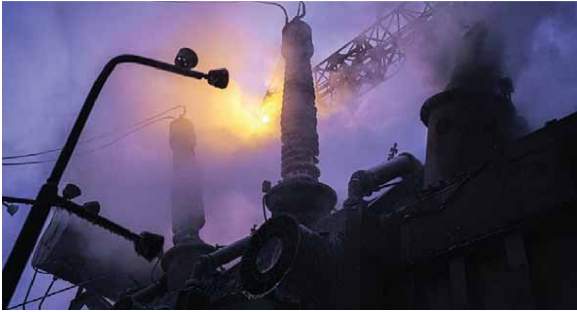
This handout picture taken and released on December 19, 2022 by Ukrainian Emergency Ministry shows a fire at a critical power infrastructure after a drone attack in Kyiv, amid the Russian invasion of Ukraine.
