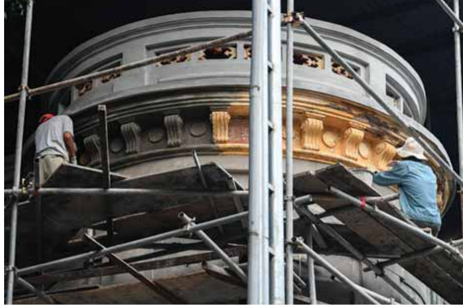
This photo shows construction workers remodeling an old villa in Hanoi.
