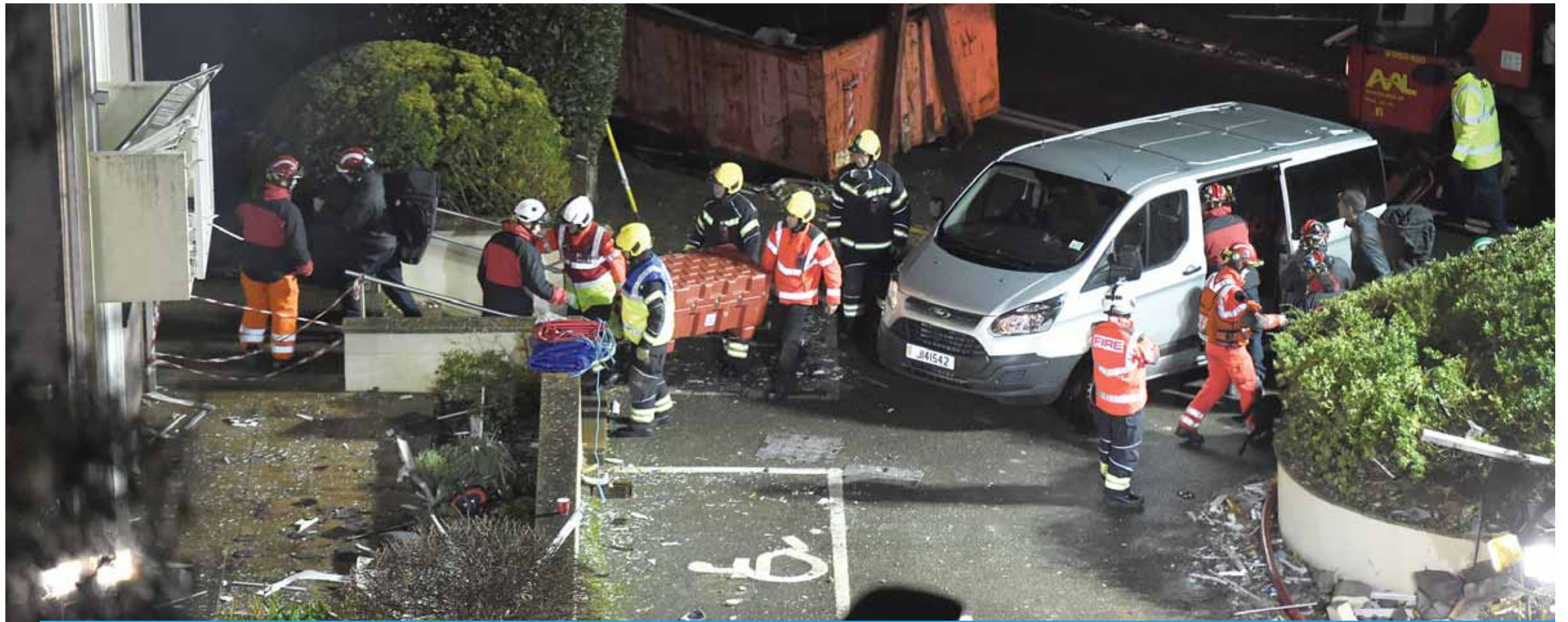
SAINT HELIER, Jersey: Fire crews mobilised work in the rubble of a low-rise apartment block after an explosion on December 10, 2022 in Saint-Helier, Jersey Island. —AFP
