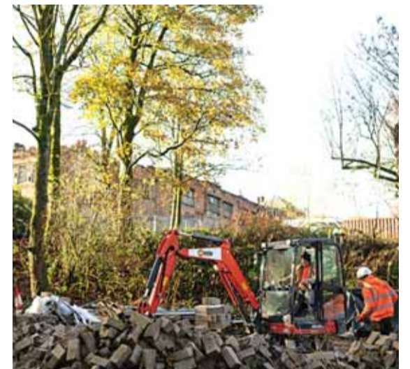
Construction workers landscape the grounds of Hopwood Hall.
