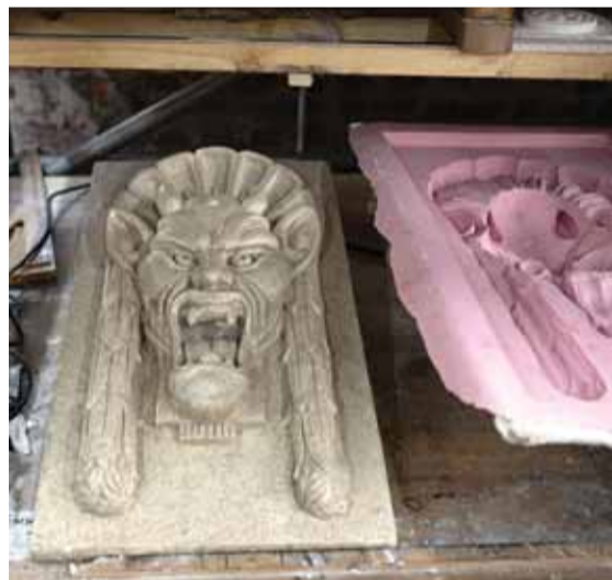
A newly-created cast that will replace the water damaged original in Hopwood Hall.
