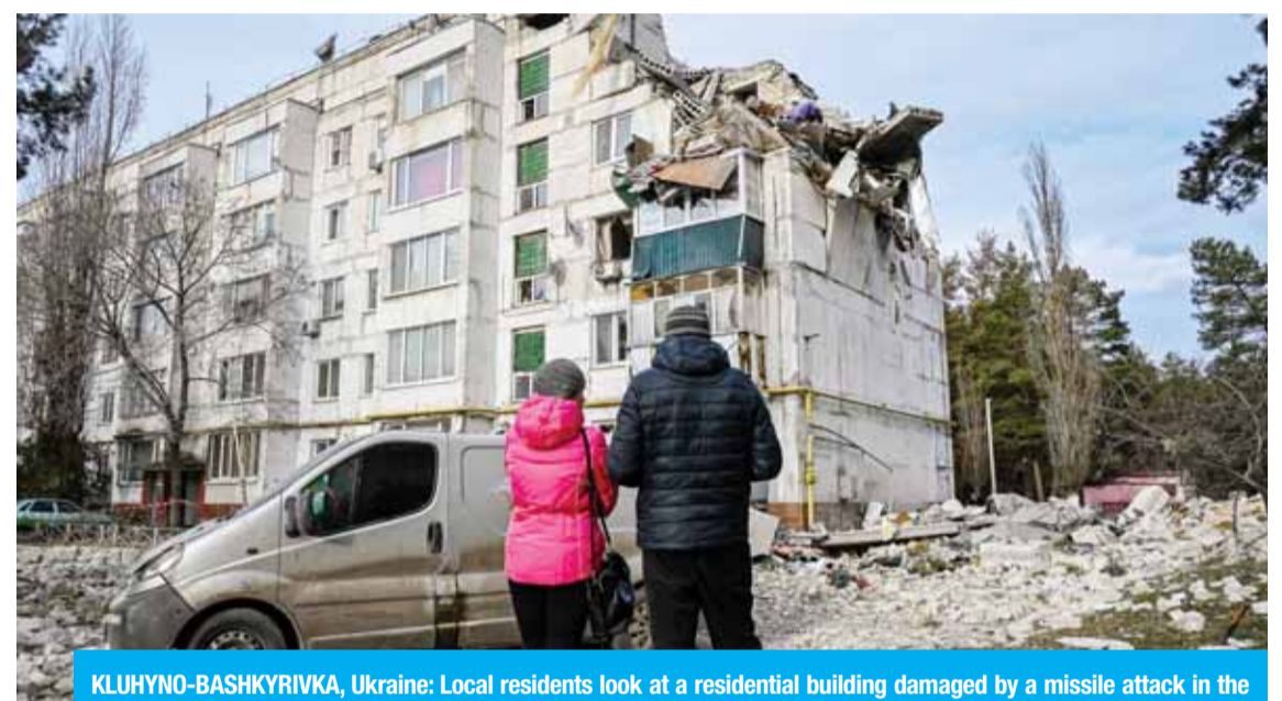
KLUHYNO-BASHKYRIVKA, Ukraine: Local residents look at a residential building damaged by a missile attack in the village of Kluhyno-Bashkyrivka, Kharkiv region, on December 2, 2022, amid the Russian invasion of Ukraine. — AFP
