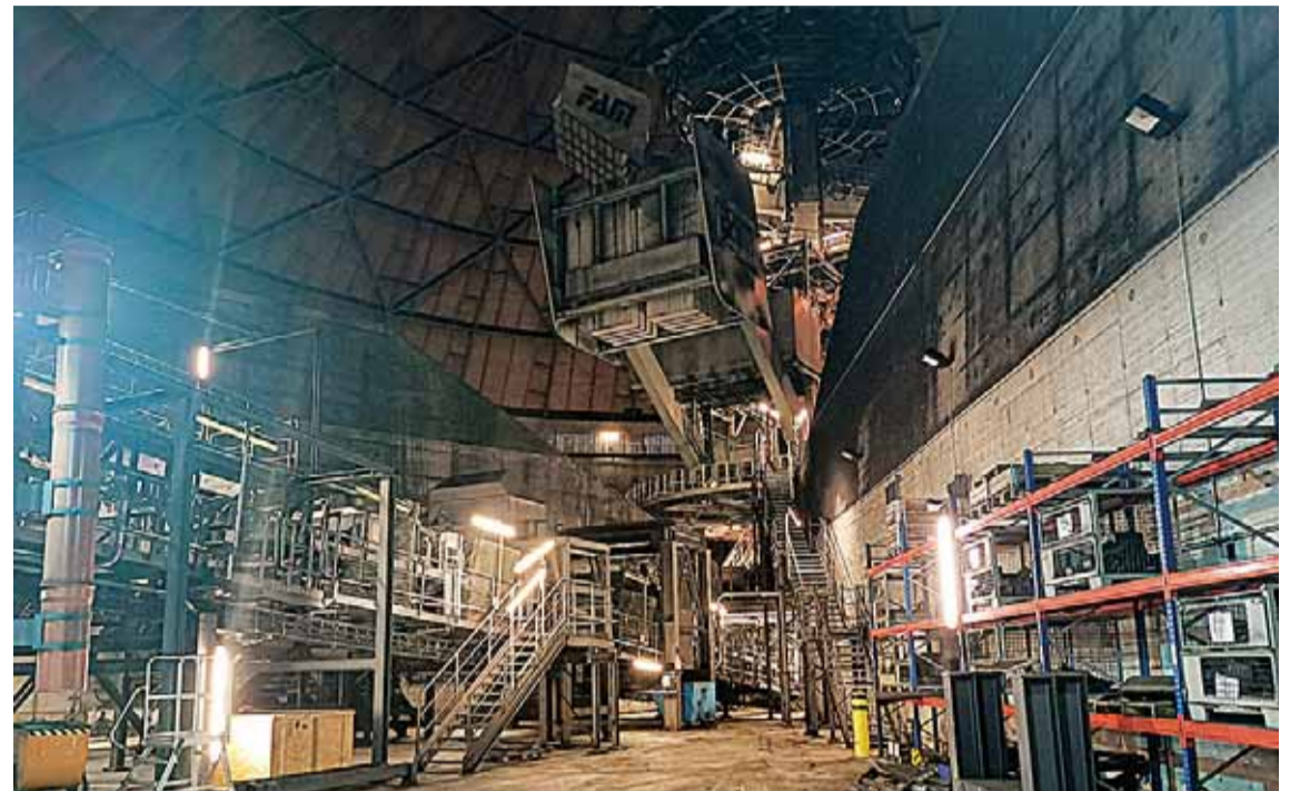
HAMBURG: This picture taken on August 25, 2022 shows the coal warehouse at the Moorburg coal power plant in Hamburg, northern Germany. —AFP
