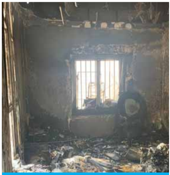
The charred interiors of a Salwa apartment.
