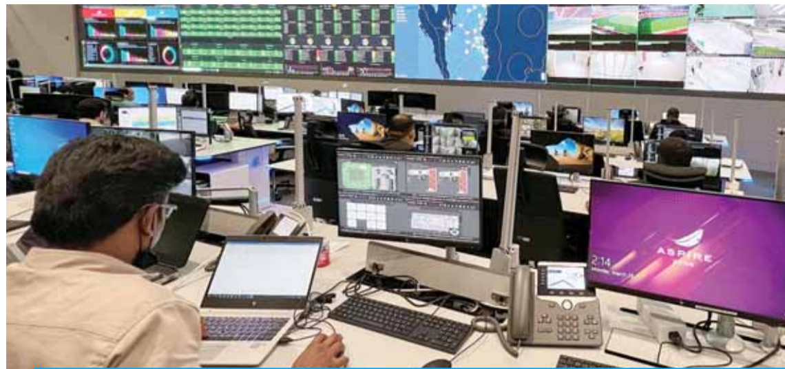
DOHA: Staff work at the Aspire security command centre for the FIFA World Cup Qatar 2022, near Khalifa International stadium in Doha, where operation and security teams will be able to monitor all the stadiums during the World Cup. — AFP
