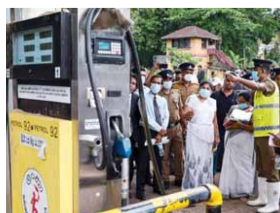
RAMBUKKANA, Sri Lanka: District magistrate Wasana Nawarathna (G) inspects a damaged Ceylon Petroleum Corporation fuel station in Rambukkana on April 20, 2022. —AFP
