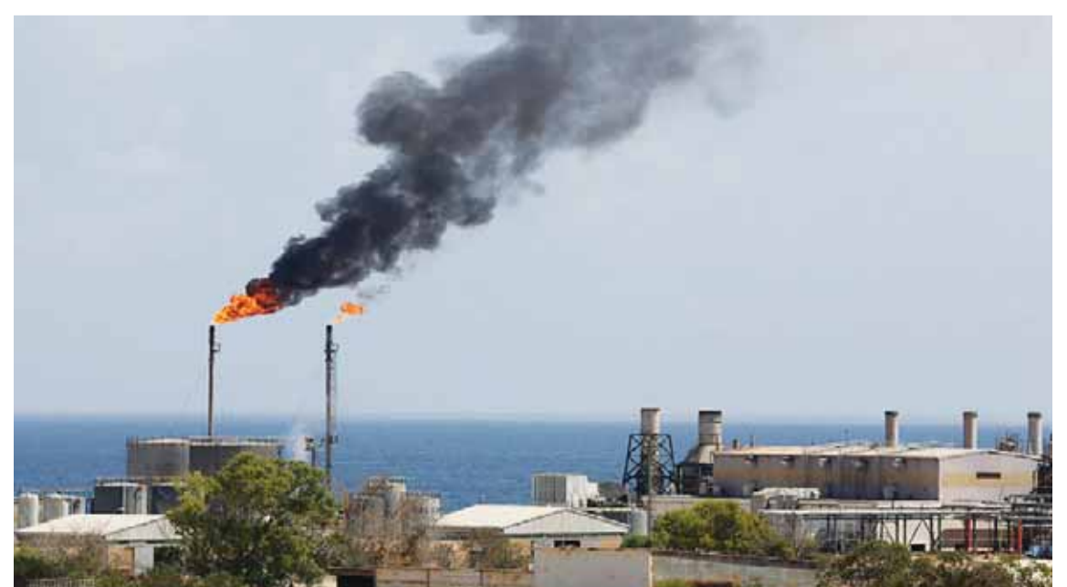
The Transmed pipeline brings gas from Algeria to Italy via this section in Tunisia
