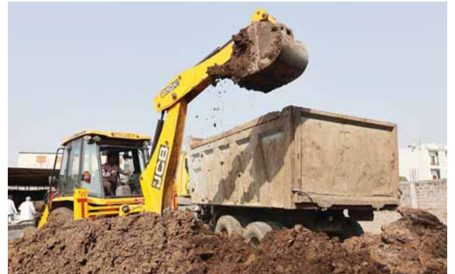
INDORE: An excavator loads cow dung for biogas production into a truck at the dairy farm of farmer Suresh Sisodia in Mayakhedi village on the outskirts of Indore.
