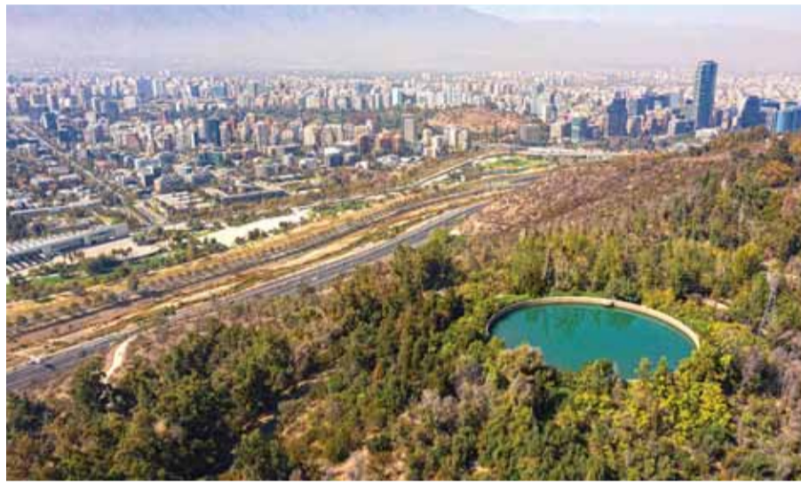
Aerial view of a water reservoir with which the Metropolitan park waters its gardens.
