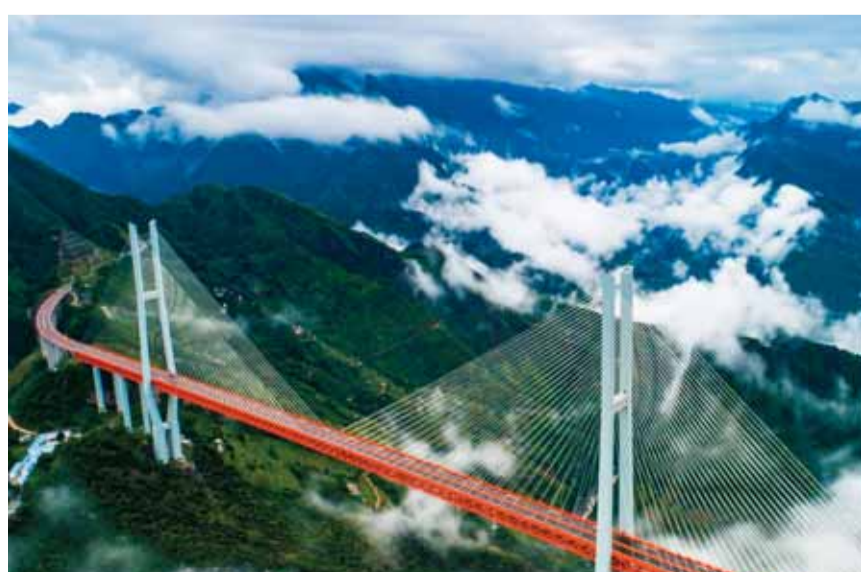
Bei Pan River Bridge in Guizhou Province, Southwest China -- The Highest Bridge in The World
