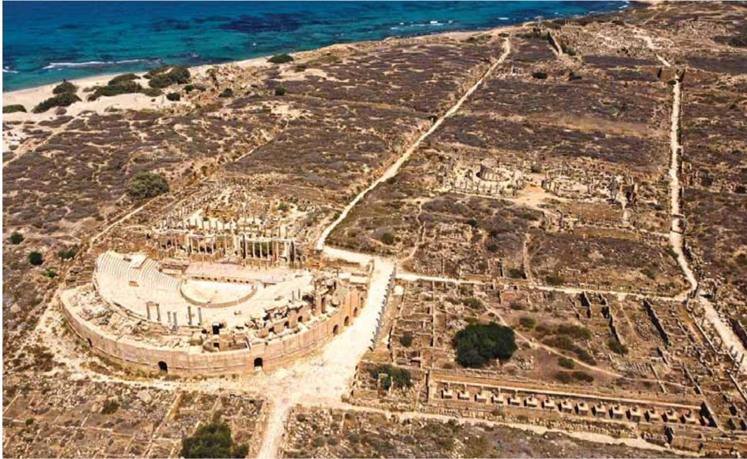
An aerial picture shows the remains of the semi-circular theatre and the Chalcidicum (right), beyond which lies the marketplace, and the Severan Forum and Basilica (top right), in the ancient Roman city of Leptis Magna near the coastal Libyan city of Al-Khums, 120Km east of the capital. -AFP photos
