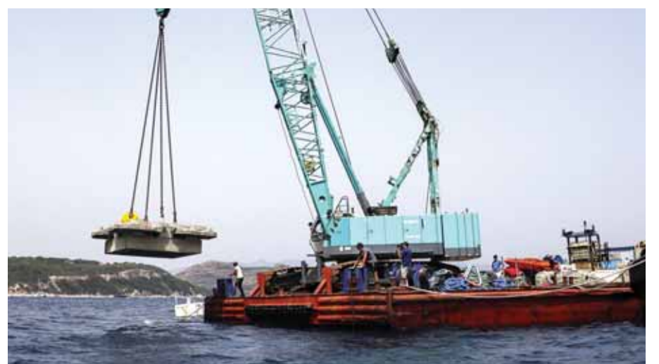
Workers immerse blocks in the sea for the anchorage of yachts in the Sant'Amanza bay close to Bonifacio in the south of the French Mediterranean island of Corsica.
