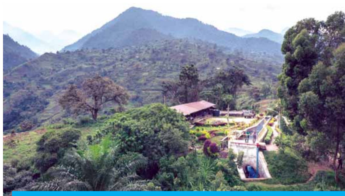
BENI: Two workers at the Mutwanga hydroelectric plant look at the facility at the foot of the Rwenzori Mountains in Beni territory, northeastern Democratic Republic of Congo. — AFP
