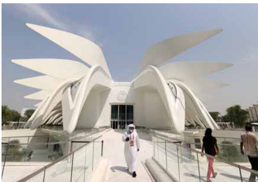
This picture shows the Emirati pavilion at the Expo 2020 yesterday.
