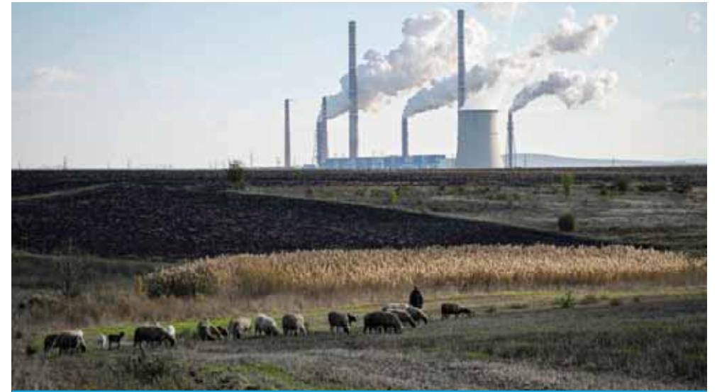
STARA ZAGORA, Bulgaria: A picture taken on October 29, 2021 shows a shepherd with his sheep in front of the Maritsa East II, the largest thermal power plant in Bulgaria. Bulgaria which joined the EU in 2007 but remains one of the bloc's poorest and also one of the most coal-dependent countries had long refrained from setting a deadline to end electricity production from coal. —AFP
