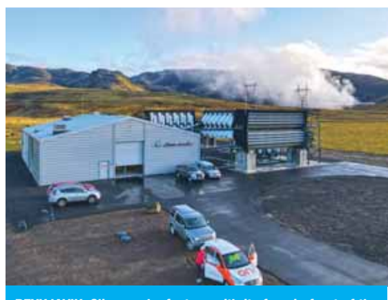
REYKJAVIK: Climevents factory with its fans in front of the collector, drawing in ambient air and release it, as largely purified CO2 through ventilators at the back is seen at the Hellisheidi power plant near Reykjavik. — AFP
