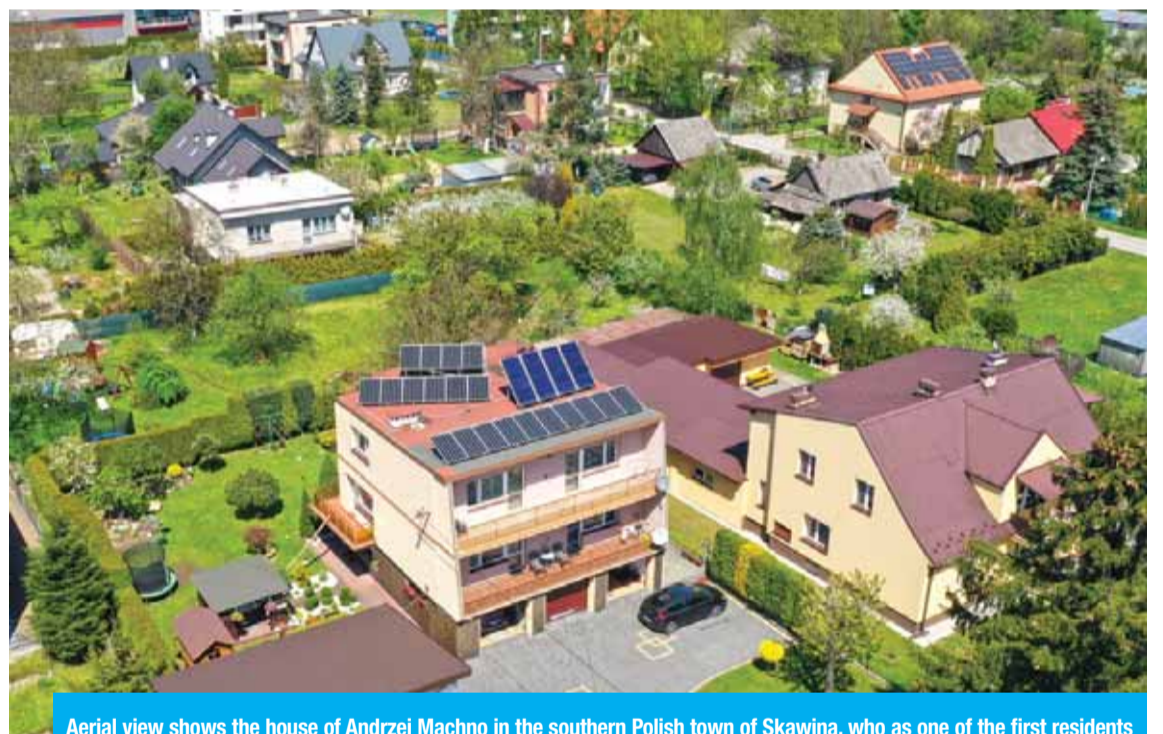
Aerial view shows the house of Andrzej Machno in the southern Polish town of Skawina, who as one of the first residents swap out his old coal boiler for solar panels. — AFP
