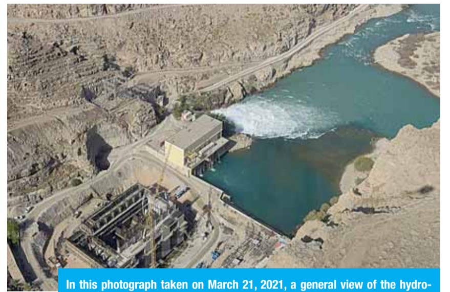
In this photograph taken on March 21, 2021, a general view of the hydroelectric Kajaki Dam is seen in Kajaki, northeast of Helmand Province. —AFP
