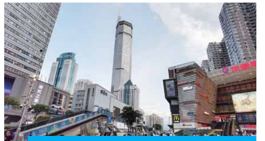
SHENZHEN: The 300-m-high SEG Plaza is seen after it began to shake yesterday. — AFP
