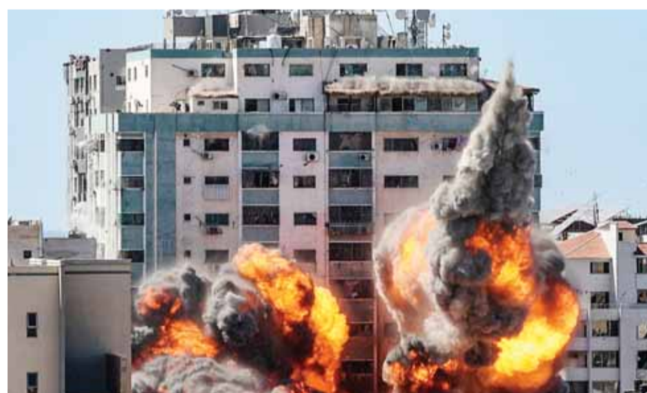
GAZA: A ball of fire erupts from the Jala Tower as it is destroyed in a Zionist airstrike in Gaza City on Saturday. — AFP
