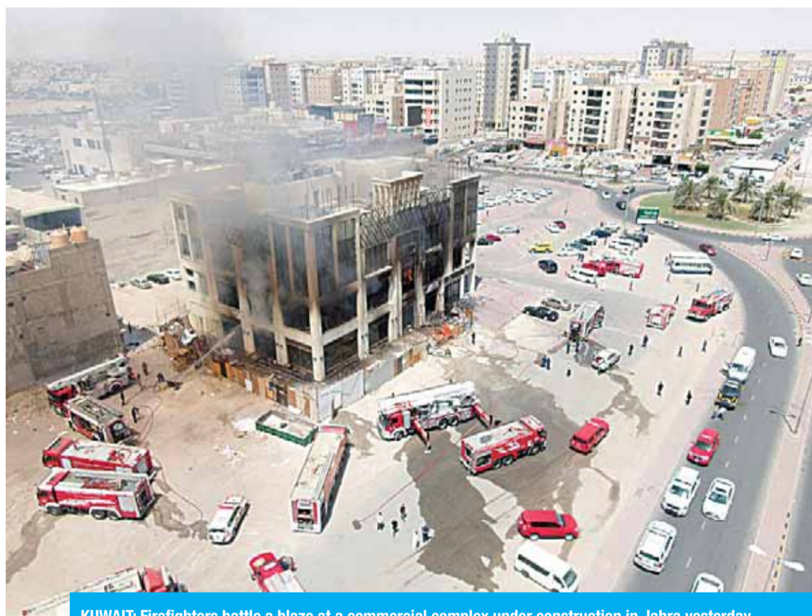
KUWAIT: Firefighters battle a blaze at a commercial complex under construction in Jahra yesterday.
