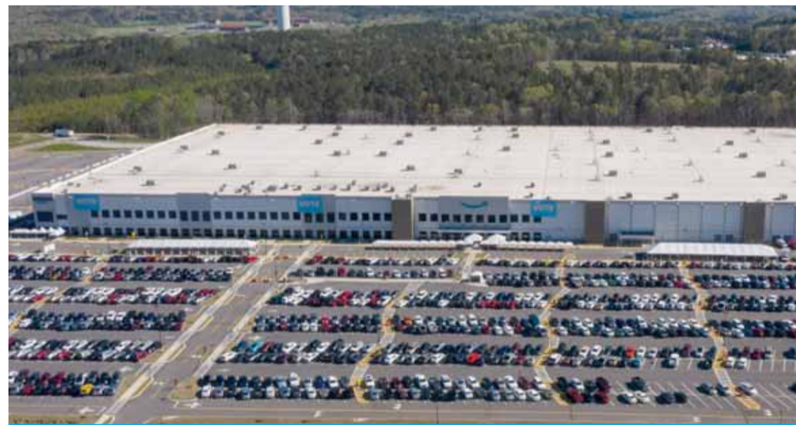
An aerial image shows the Amazon.com, Inc BHM1 fulfillment center on Monday in Bessemer, Alabama.
