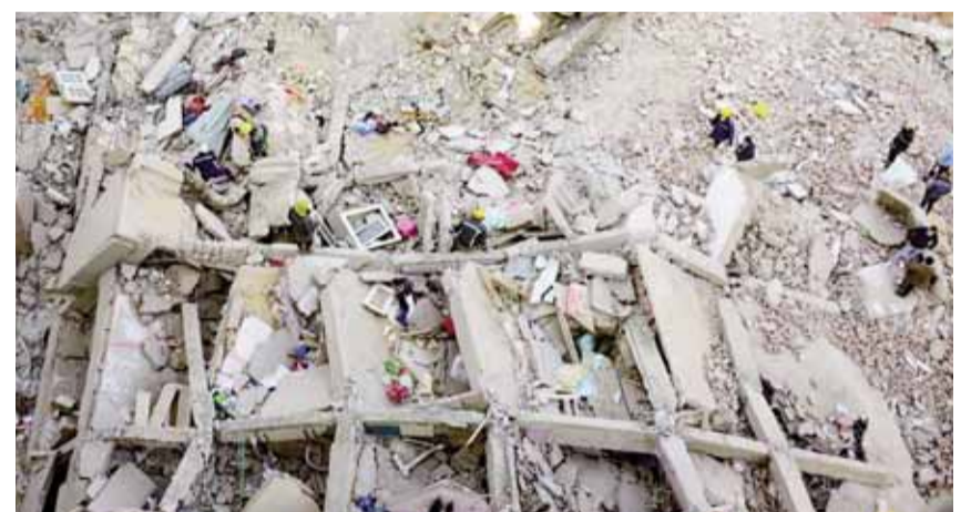
CAIRO: People and rescuers gather around the rubble of a building that collapsed in Gesr Suez, east of the Egyptian capital, on Saturday. — AFP
