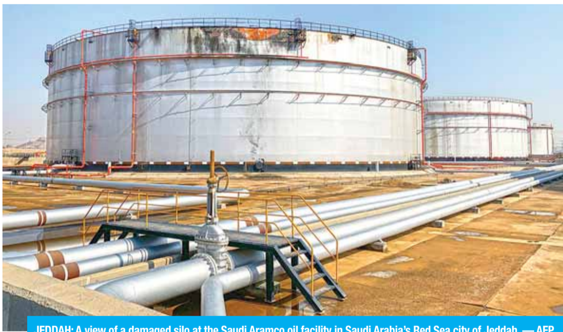
JEDDAH: A view of a damaged silo at the Saudi Aramco oil facility in Saudi Arabia's Red Sea city of Jeddah. — AFP
