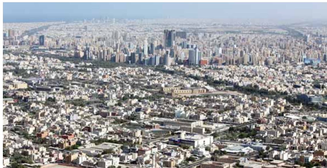
KUWAIT: A general view of buildings in Kuwait City and its surrounding areas in this archive photo. —Photo by Yasser Al-Zayyat
